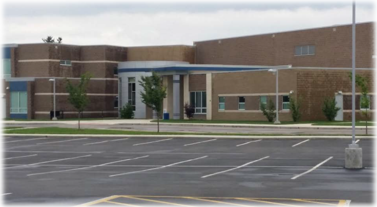
The photo above is a representation of the appearance of all five new elementary buildings
